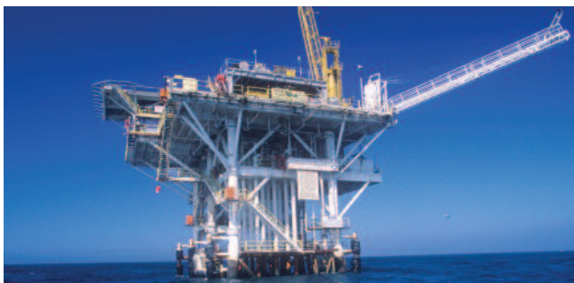
Offshore / Civil Marine
